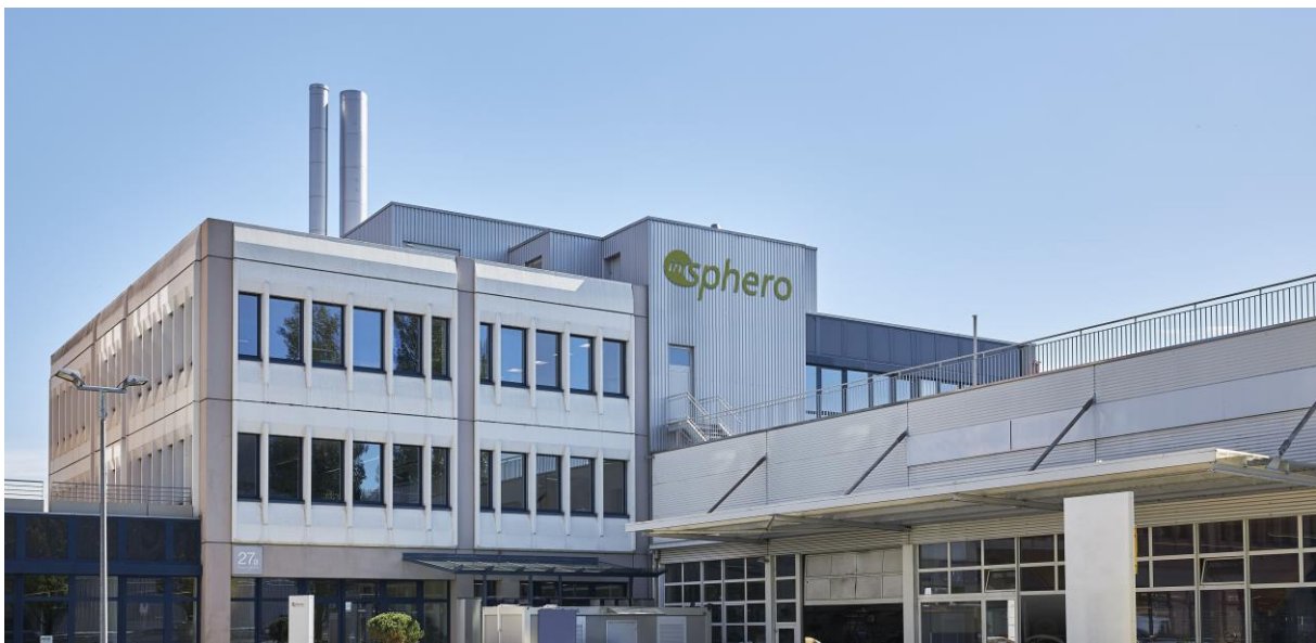
InSphero's new corporate headquarters located at Wagistrasse 27A, Schlieren, Switzerland.
